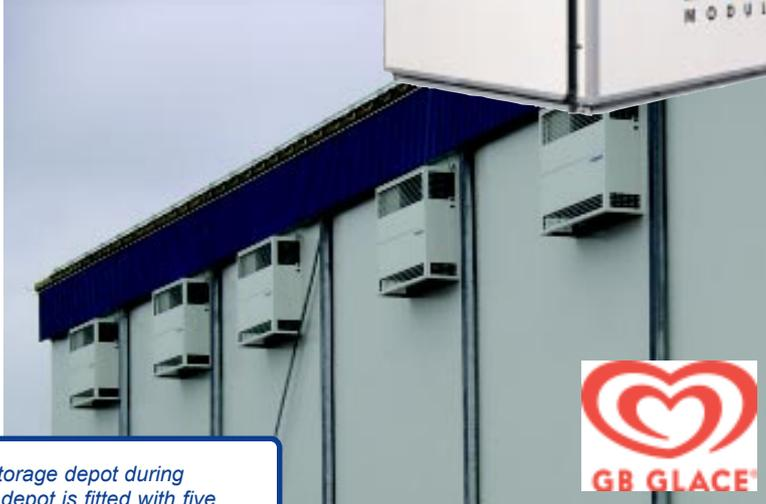
*Large ice cream storage depot during construction. This depot is fitted with five Megafrost-110-V plug-in units to BoxModule's specification (Total 40 kW at -28°C room temperature)*
