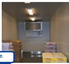
*11 kW cooler unit installed in small cold storage module.*
